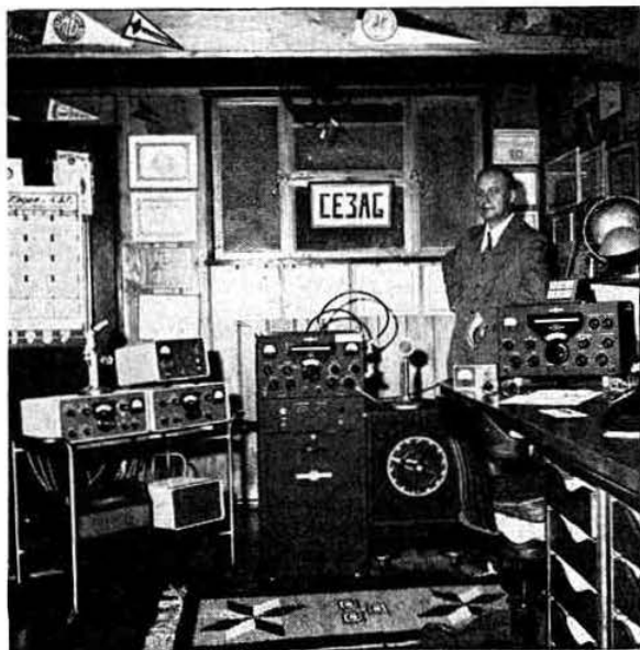
CE3AG uses the Collins equipment shown in this picture with a 3-element tri-band "W3DZZ" beam for 14, 21 and 28 Mc/s. He has worked 286 countries and has 285 confirmed. Operation is principally on c.w. and s.s.b.
